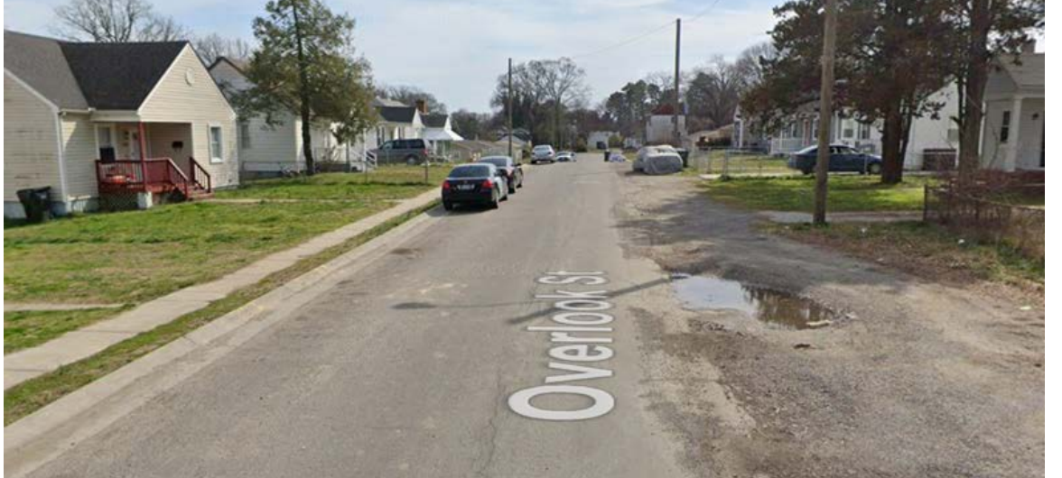
Lack of sidewalks in Bellemeade/Oak Grove
