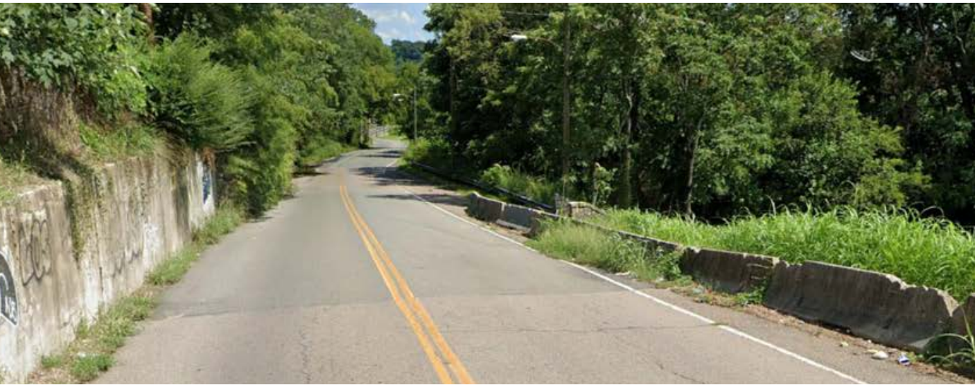
Sidewalks lacking along Williamsburg Rd
