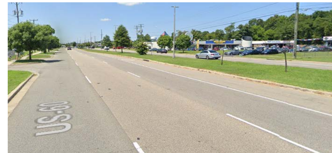
Unsafe pedestrian environment on Midlothian Tpke
