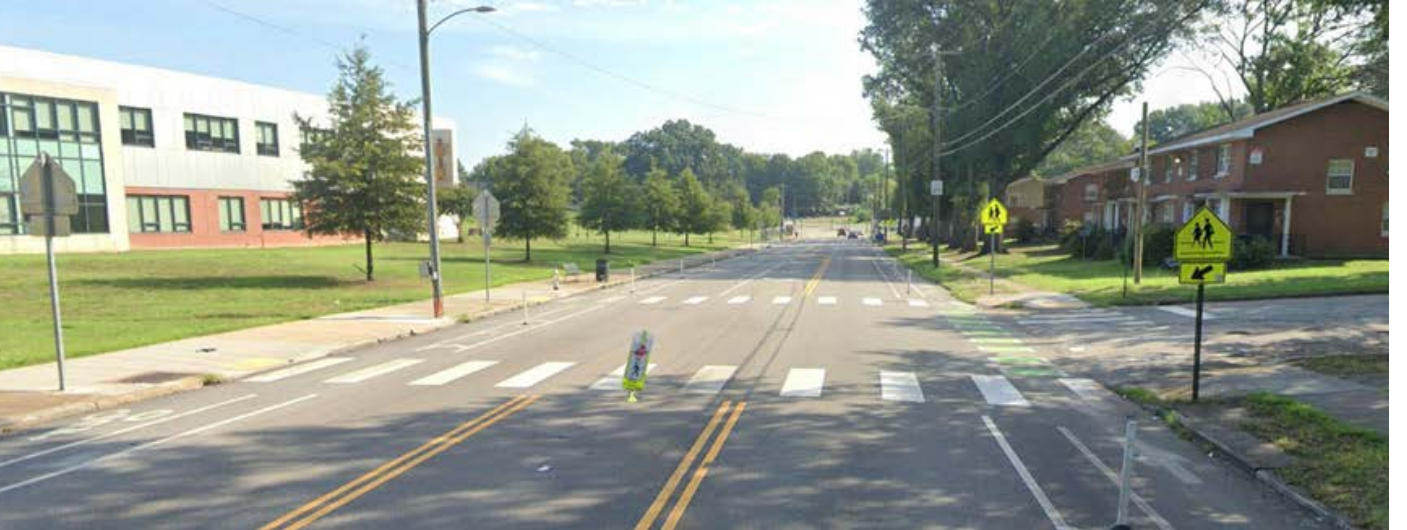
Pedestrian crossing facilities on Mosby St at MLK Middle School
